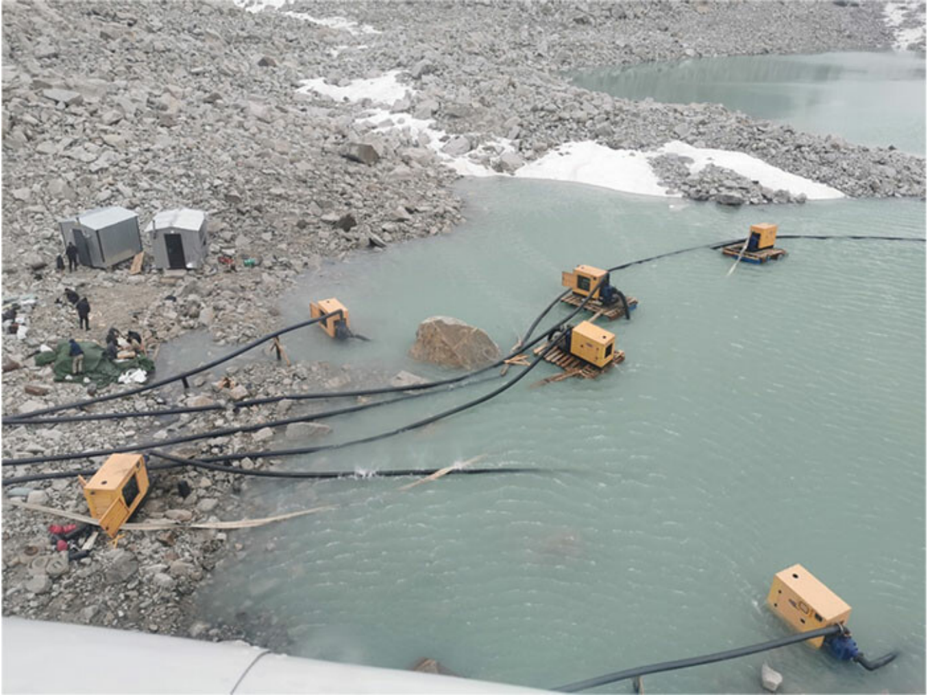
Figure 3. Drainage of lake No. 13 through a pumping system in the Ulken Almaty River catchment of the Kazakh Ile Alatau.
