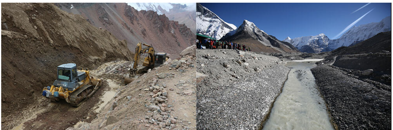
Figure 4. Left: Clearing and deepening of a surface drainage channel from lake No. 6 in the Kishi Almaty River catchment of the Kazakh Ile Alatau. Right: Surface drainage channel at Lake Imja in Nepal.
