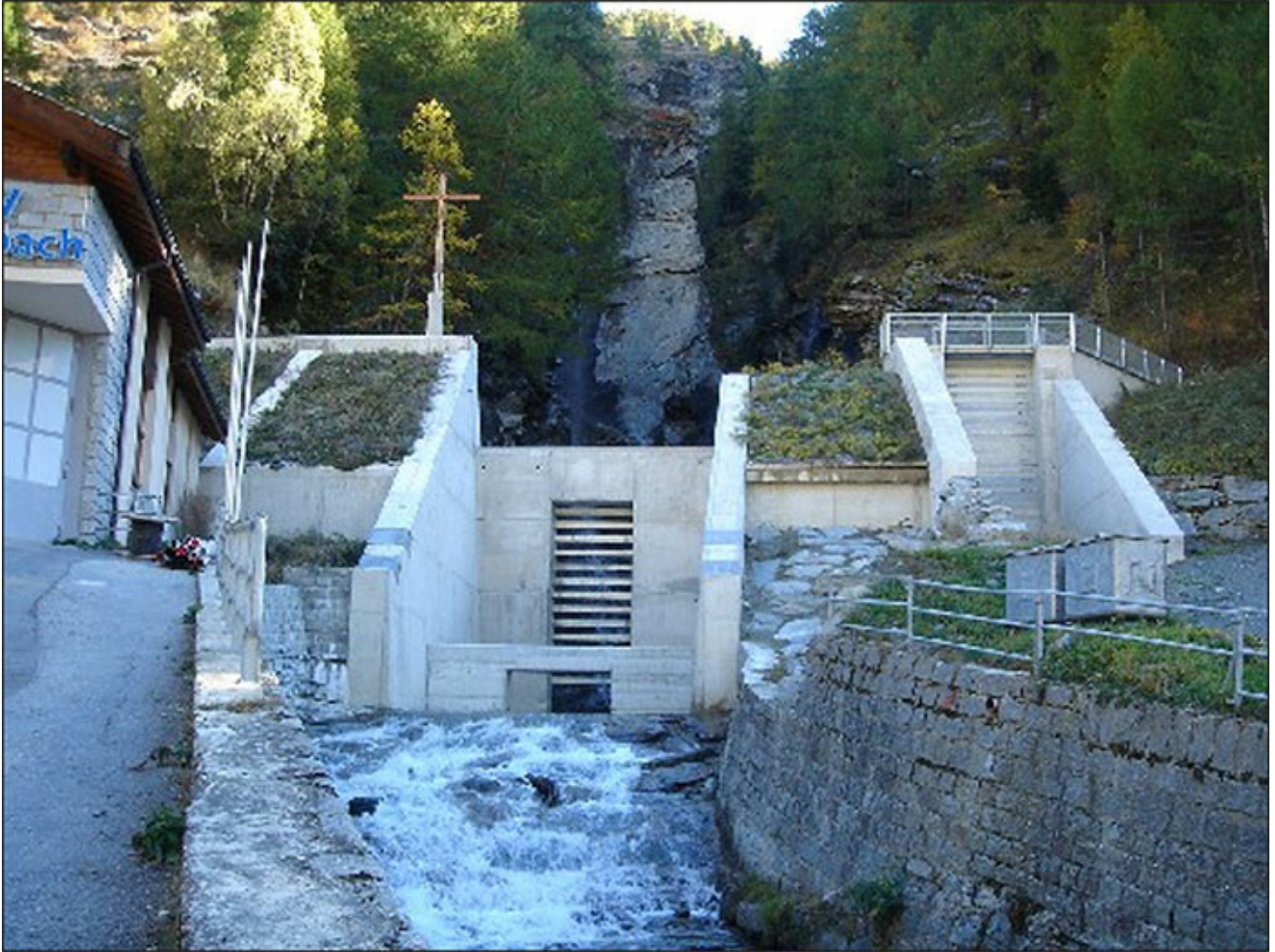
Figure 6. Sediment retention structure in Täsch, downstream of lake Weingarten in Switzerland.
